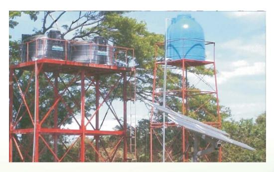
Large Stationery PV Water Pump with Tracking System. With the tracker the solar water pumping system can harness the sun's power efficiently and provide more energy in areas of low solar irradiation.
