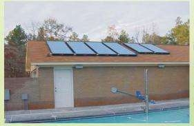
Pool heating is a very good solar application. The systems are simple and relatively inexpensive. The pool itself is the thermal storage for the system, and the pump you already use for filtering pool water will also circulate water through the solar collectors.
